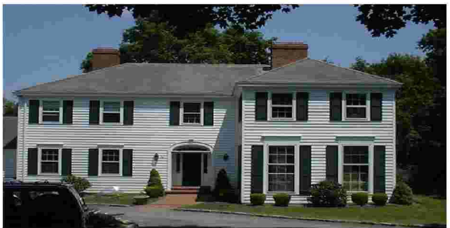
The roof on the house pictured above is covered with Transite roofing shingles, which contain Asbestos. From a distance this roof looks like any ordinary roof. In order to determine material content, a sample must be analyzed by a licensed lab.
