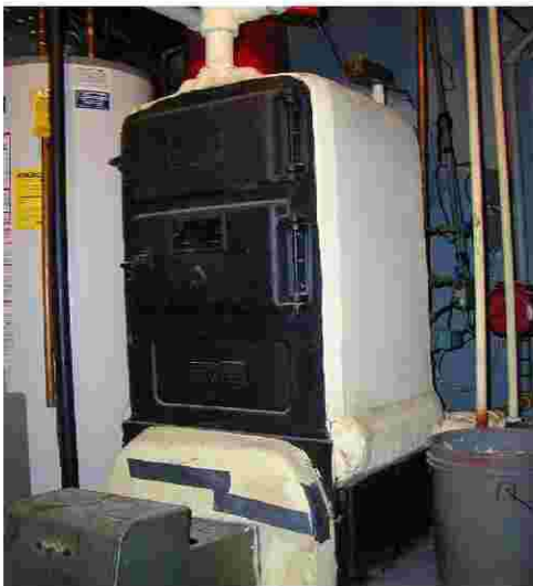
A typical boiler covered with Asbestos Cement
